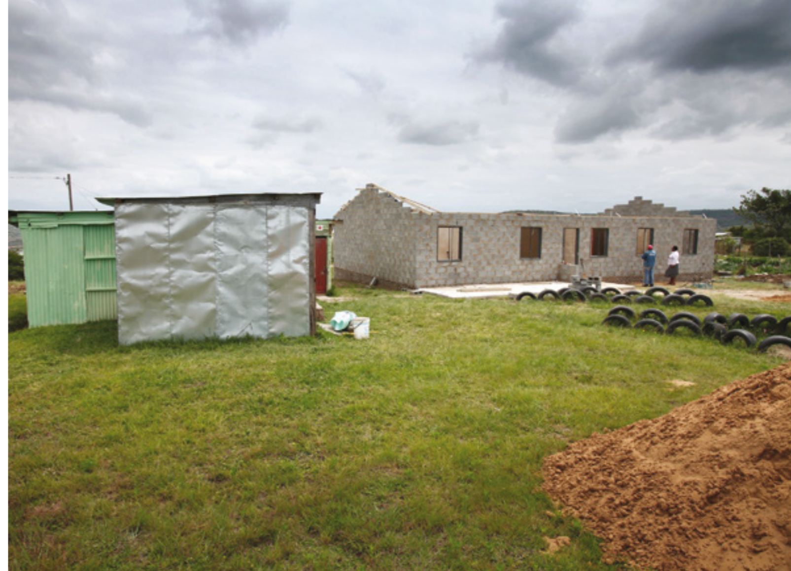
Construction at Khanya Education Centre
