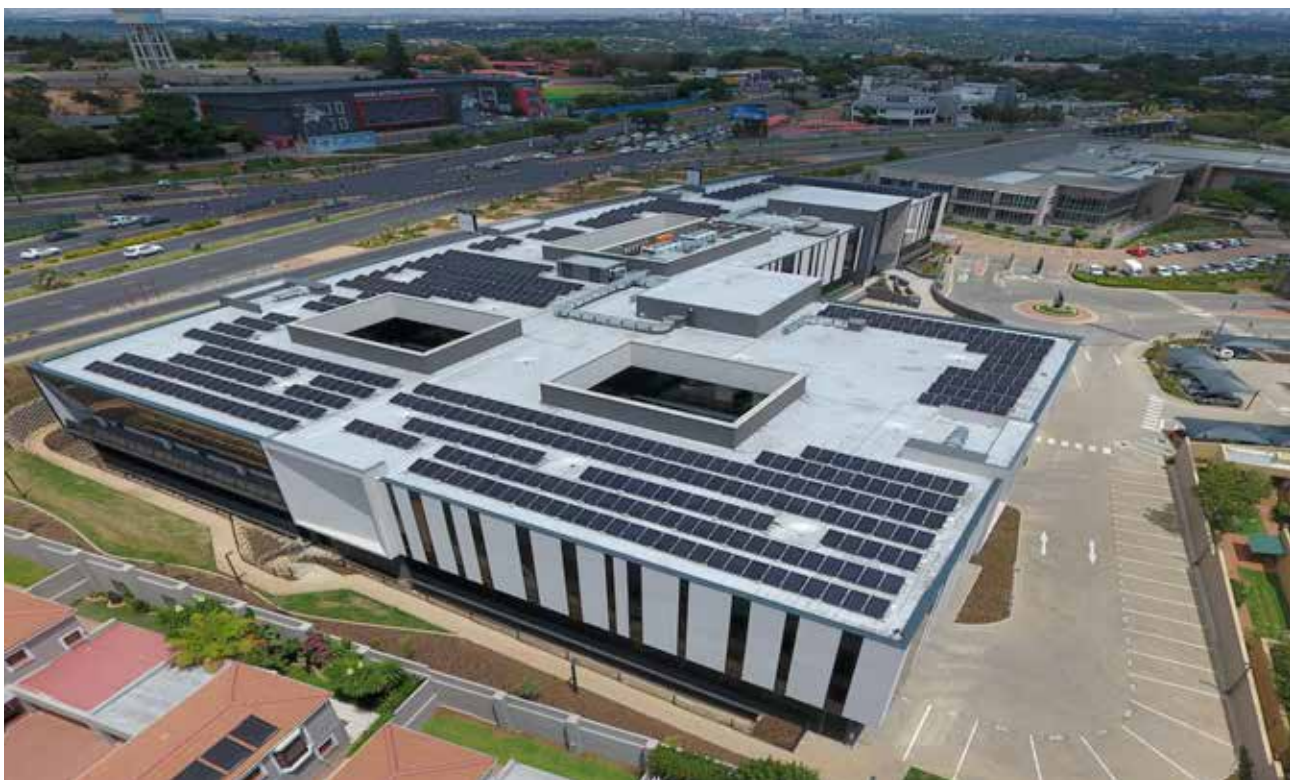
Solar panels at Anslow, Bryanston
